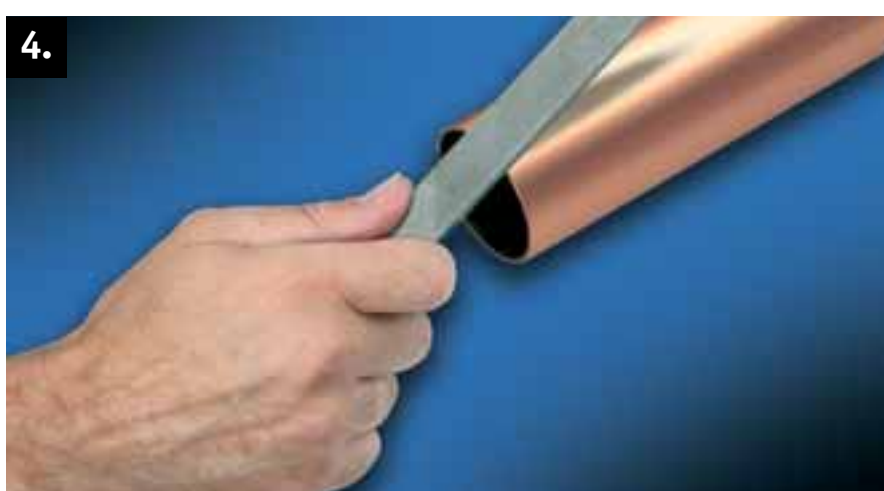
4. If a deburrer is not available use a fine file to prepare the tube end.
