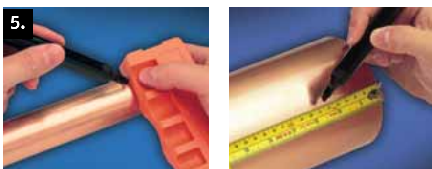
5. The tube must be fully inserted to the fitting until it meets the tube stop. Use a S110 XPress depth gauge or ruler to mark the insertion (socket) depth of the fitting onto the tube – see table below.
